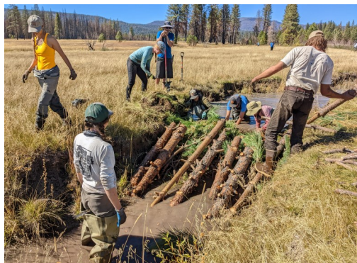
Participants in the Fall 2022 Cal PBR training construct low-tech structures in portions of Yellow Creek. Photos by Carrie Monohan, The Sierra Fund.
