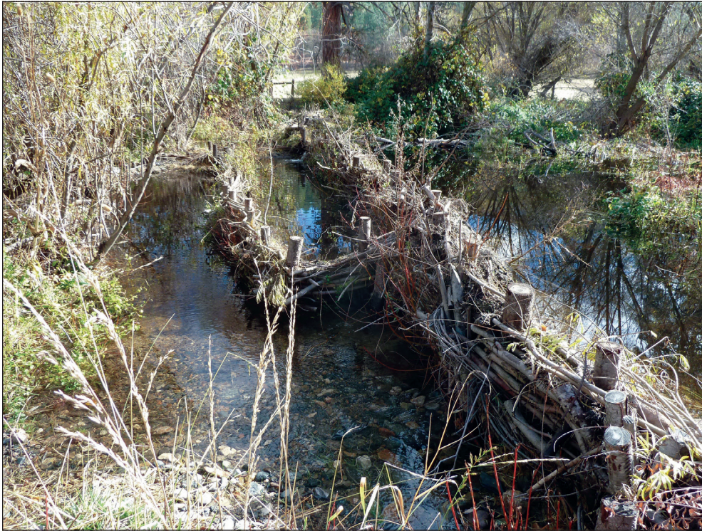
Figure 3—A beaver dam analogue constructed in Miners Creek.
