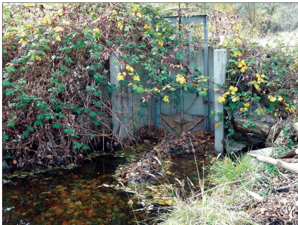
Figure 9—A V-shaped wire structure keeps beaver from plugging a water diversion into an irrigation canal.
